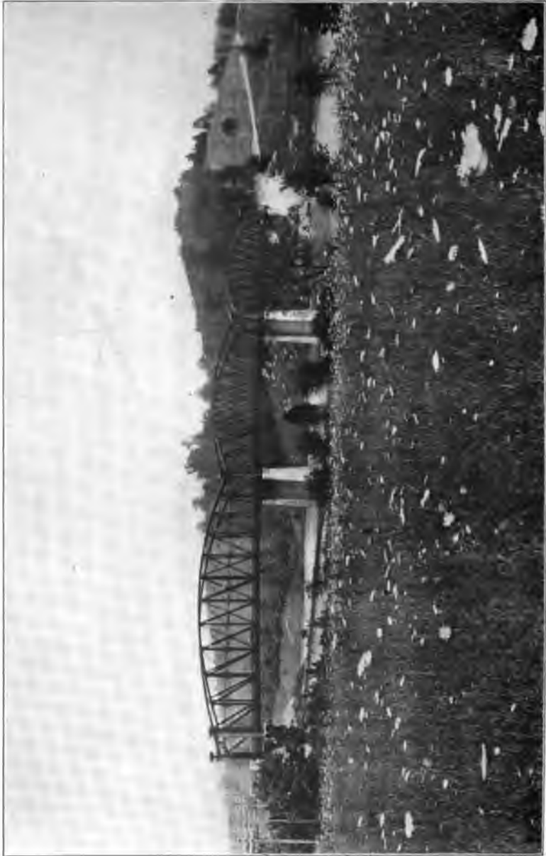
Fig. 158. Lock Raven Highway Bridge No. 2 of the Baltimore City Water Department, Baltimore, Md. The Parker trusses have a span of 297 feet, and are supported near the tops of the steel towers. Erected in 1914.
